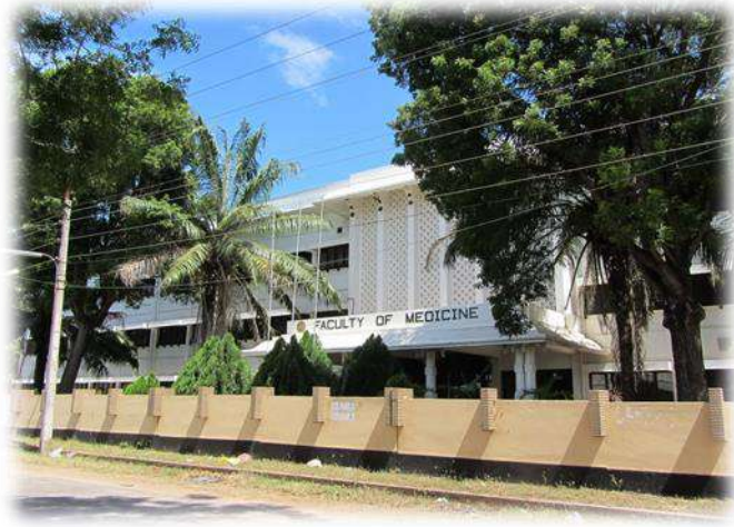
Figure 2. Entrance to the Faculty building
